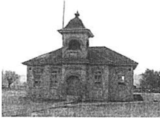
Fairfield School House, 1898
